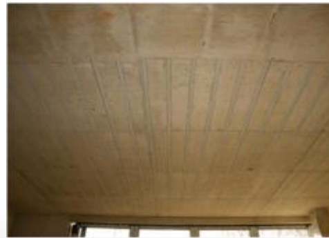
Acoustic wave breakers in thermally active concrete
