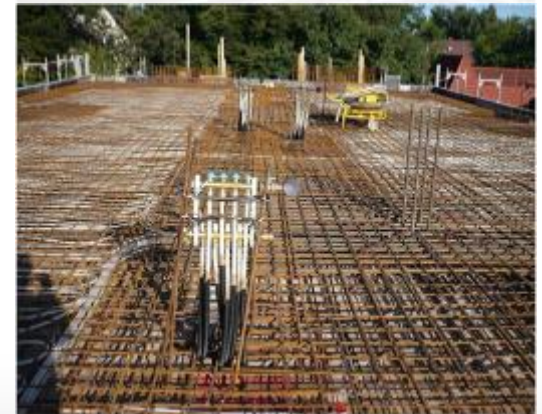
Example: inHaus2 – concrete core activation
